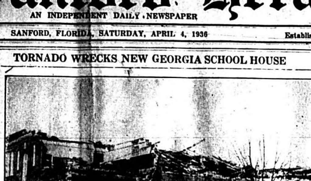
This new high school building was practically destroyed when a tornado ripped through Gordo, Ga., killing 16 persons and injuring 1,000. Hundreds of dwellings, among which were some of the city's finest, also were razed by the twister. (AP Photo)
