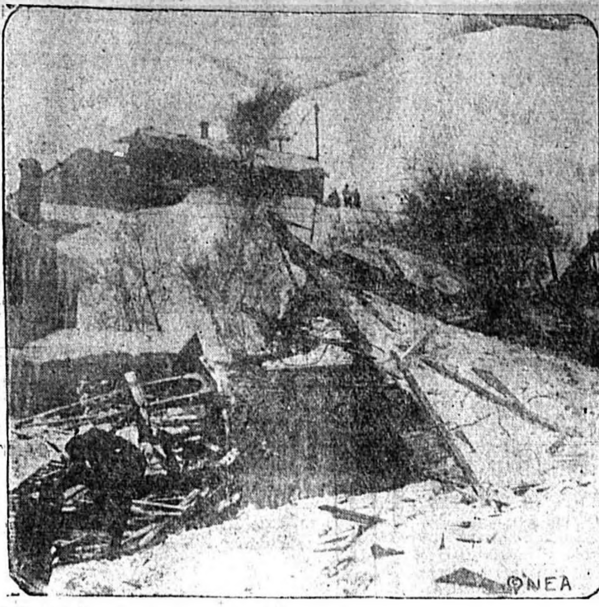
The area here destruction dealt homes which were in the path of the San Gulch, Utah, snowslides again Feb. 19. Buildings were buried under a foot of snow, and the town completely buried without warning of the disaster, dozens of persons met death.
