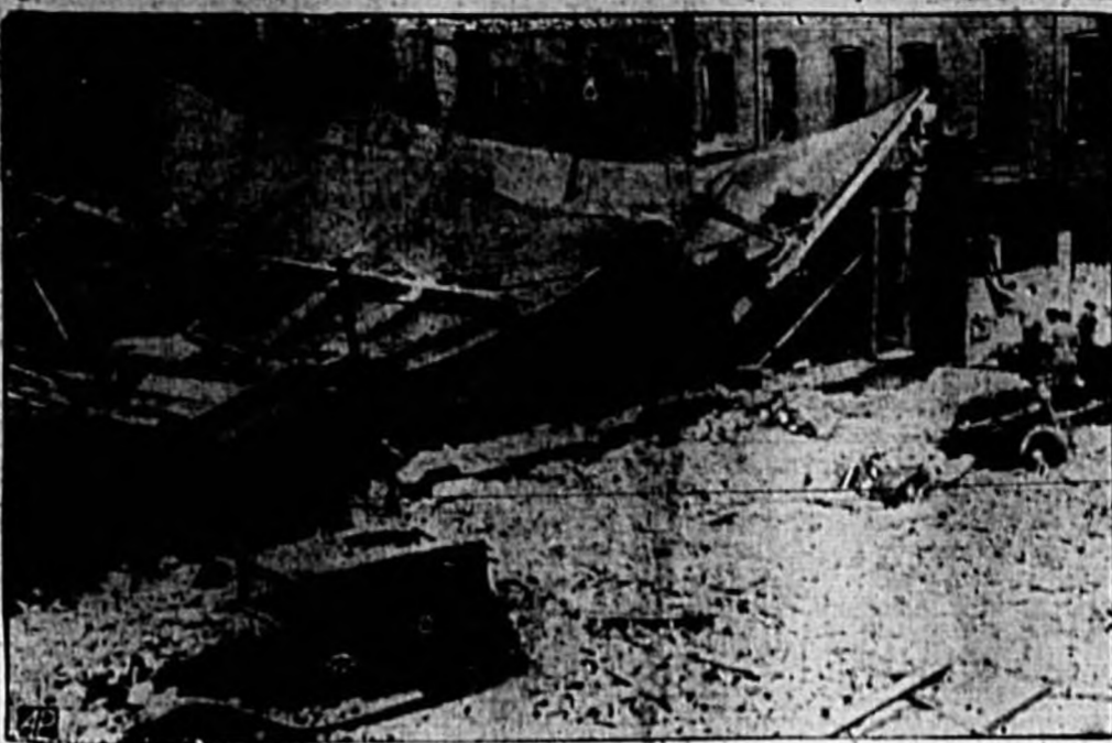
At least one person was killed and 40 others were injured in a terrific explosion that demolished a brick factory at Paterson, N. J. Houses were jarred for blocks around. The blast was believed to have originated in a gas oven. The wreckage of the building is shown shortly after the explosion. Note the automobiles partially buried under debris.
