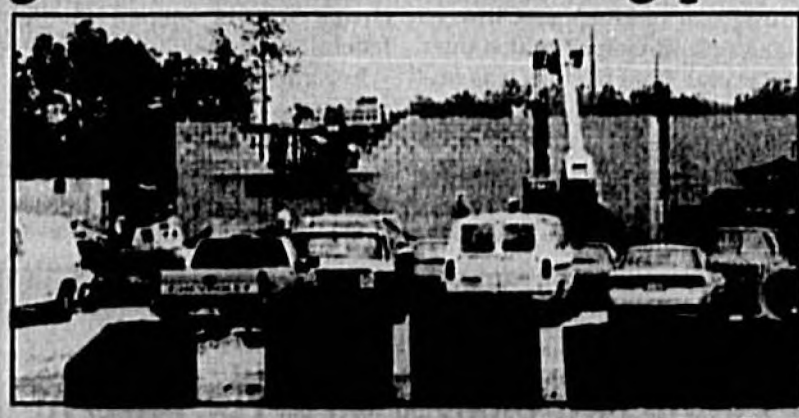
Work continues on Lawton Chiles Middle School.
