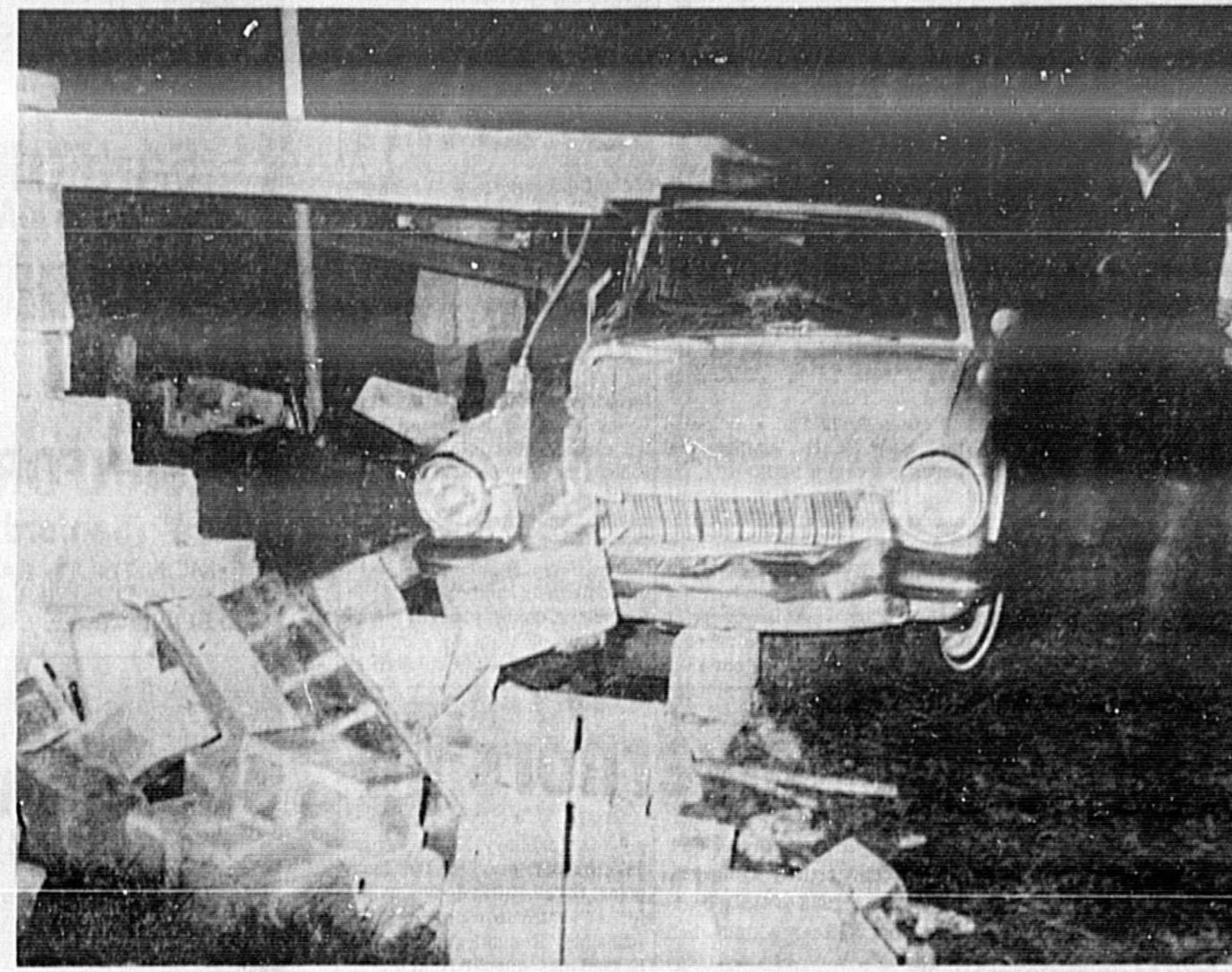
AND THE BLOCKS CAME TUMBLIN' DOWN PUMP HOUSE owned by the City of Sanford was destroyed Friday night when a car driven by Mary Ann Hopkins of Longwood slammed into the cement block fixture located in the median on Highway 17-92. The house was extensively damaged and the car was listed a total loss, according to Trooper Tommy Tomlinson, investigator. The woman was treated for cuts and bruises at Seminole Memorial Hospital and released. (Staff Photo)
