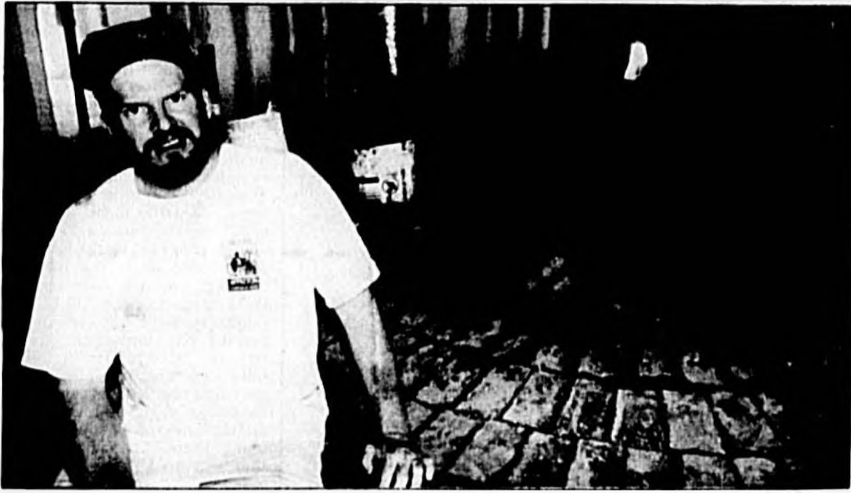
Shannon Tally, owner and master baker, assists Manuel del la Rosa with the installation of the Llopis oven. The oven was built in Spain at a cost of $50,000. Installation at the bakery was over seven days.
