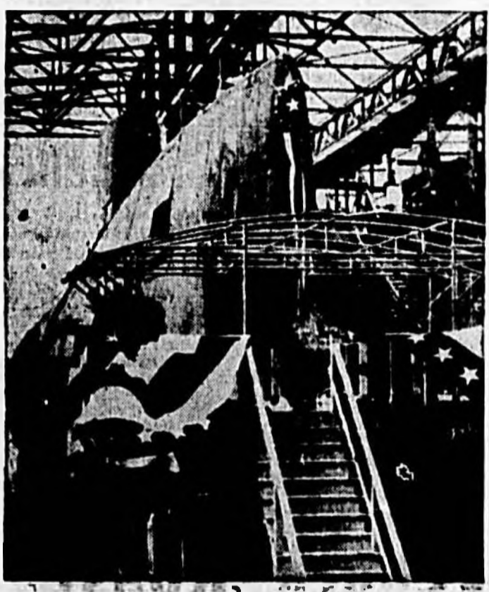
SHORTLY BEFORE being launched at the electric boat division in Groton, Conn., the submarine Darter is draped with bunting over the bow by workmen hampered by stormy weather. This latest undersea craft will be equipped with airplane-type controls. (International)
