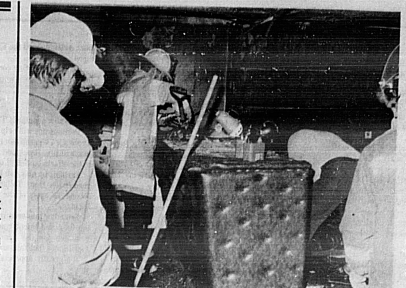
Fremmen clear damaged clubhouse while investigator, right background, probes area where blaze apparently started
