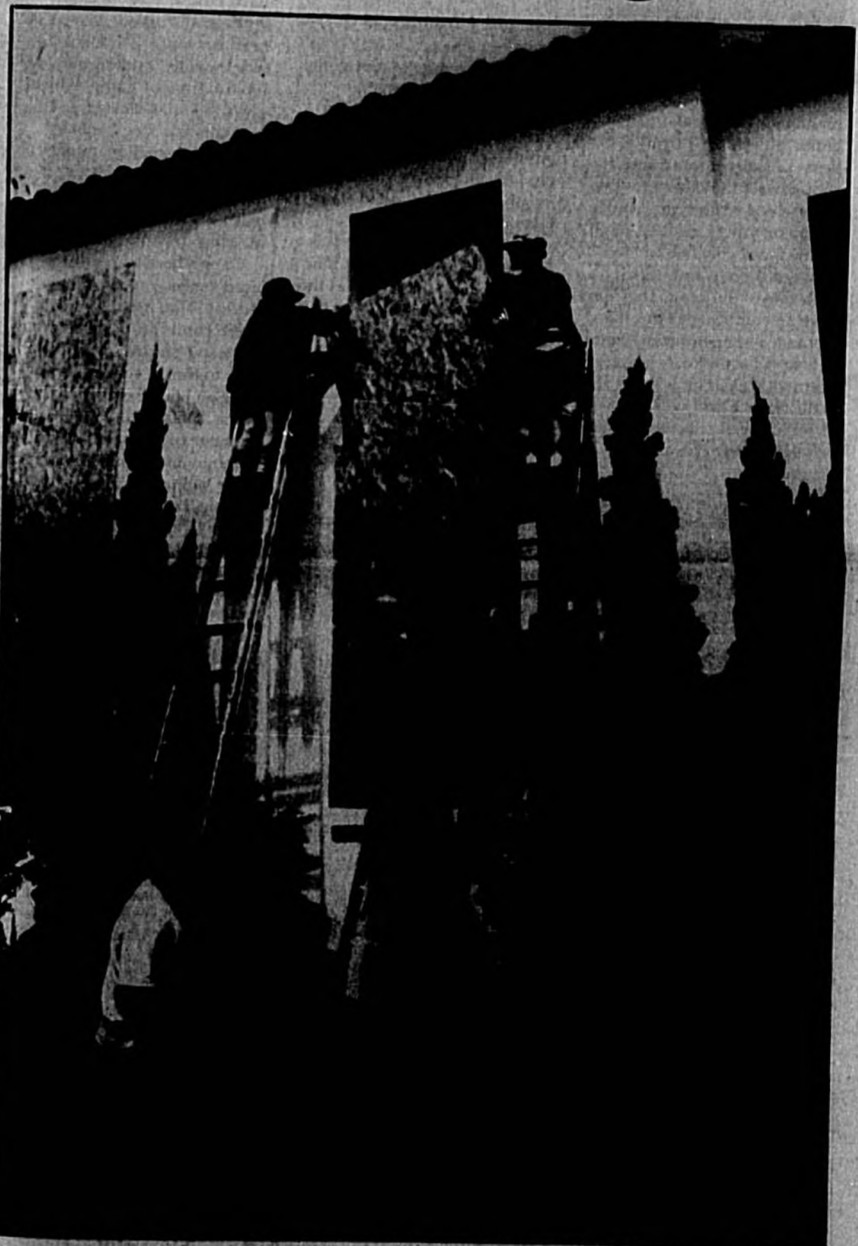
Herald photo by Tommy Vincent Frank Liberatore, Brian Brooks, Tom Gery and an unidentified worker secure plywood over the stain-glass windows at All Souls Catholic Church in Sanford.
