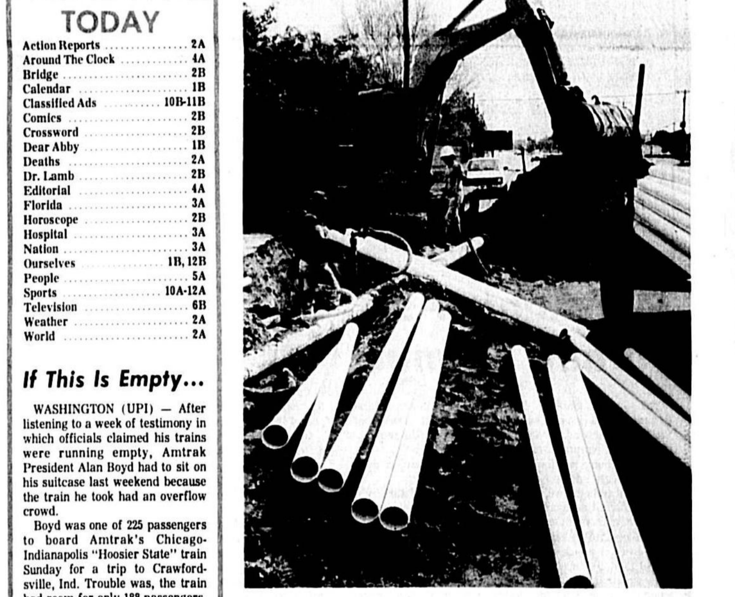
GOING UNDERGROUND Southern Bell crews have begun work on a $114,000 project along State Road 46 west of Sanford in which several miles of aerial telephone cable will be laid underground...
