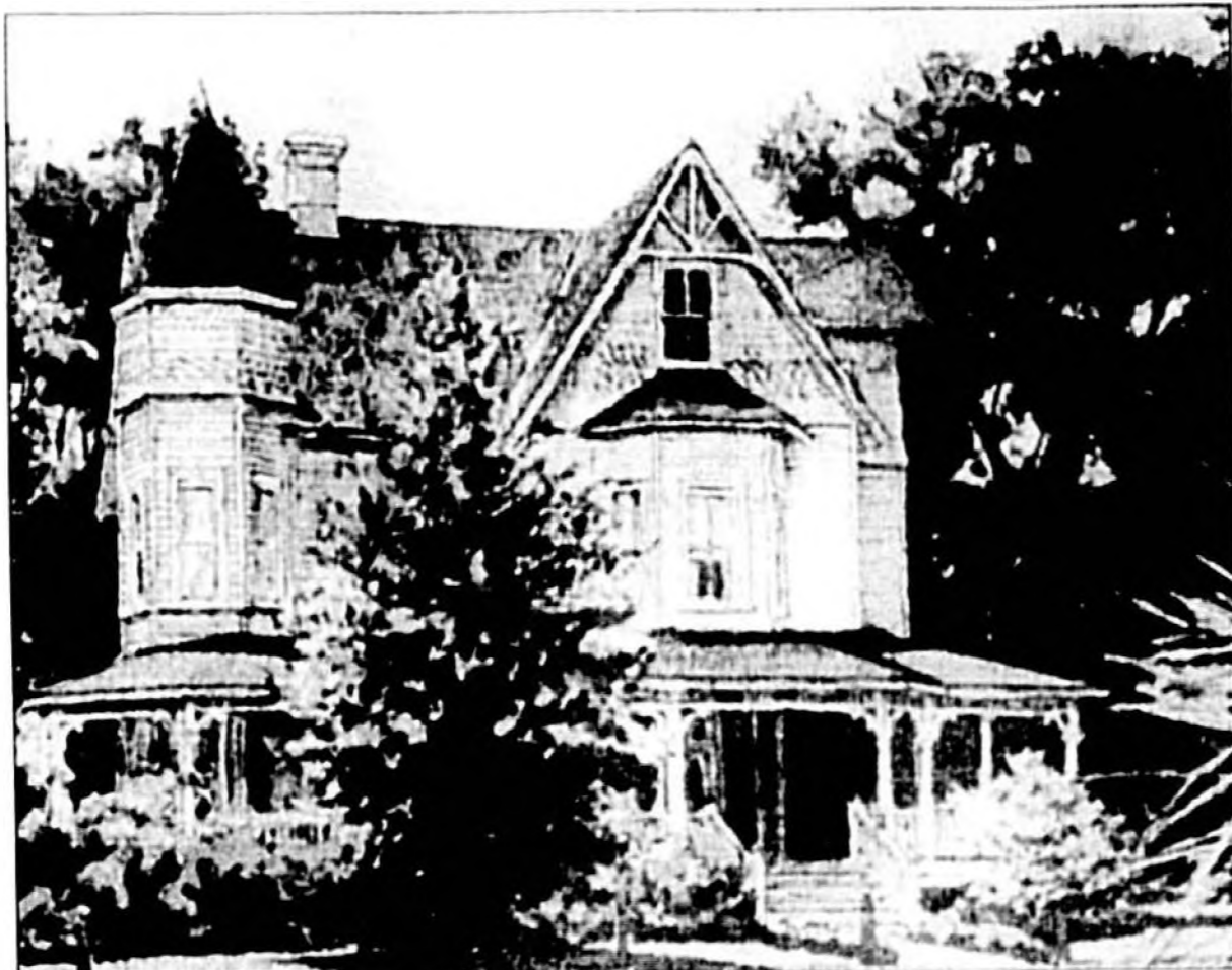
along Church and Warren avenues.
