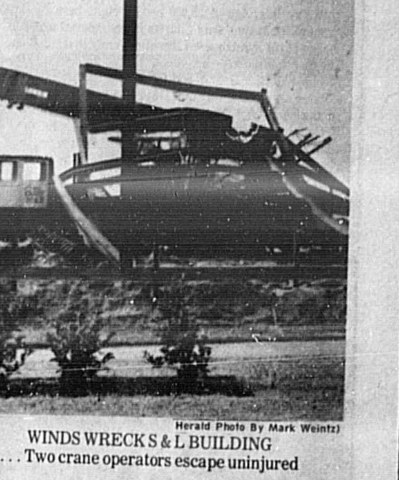
WINDS WRECK S & L BUILDING Two crane operators escape uninjured
