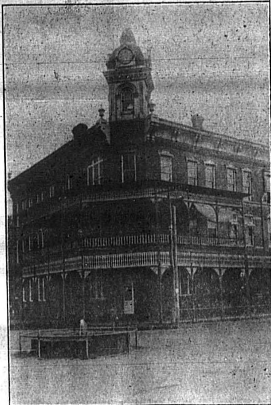
SEMINOLE BANK BUILDING
