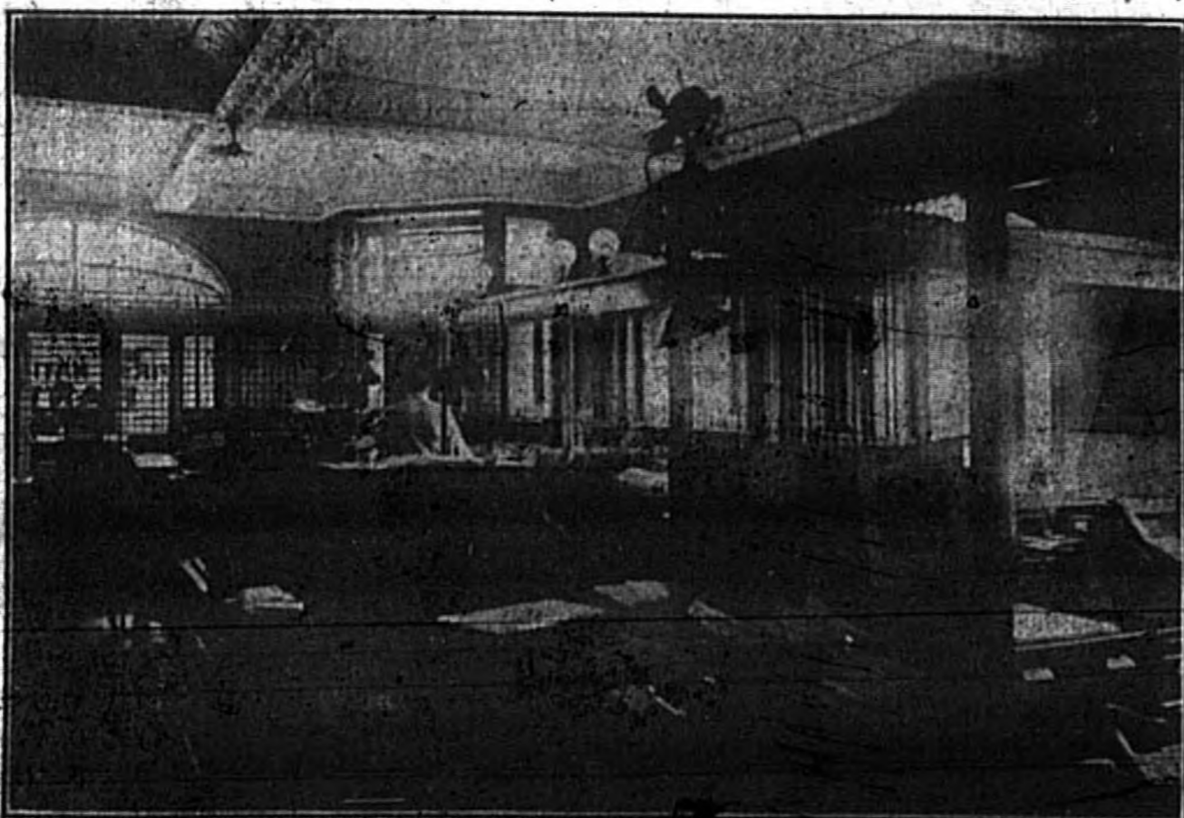
INTERIOR VIEW IN FIRST NATIONAL BANK
