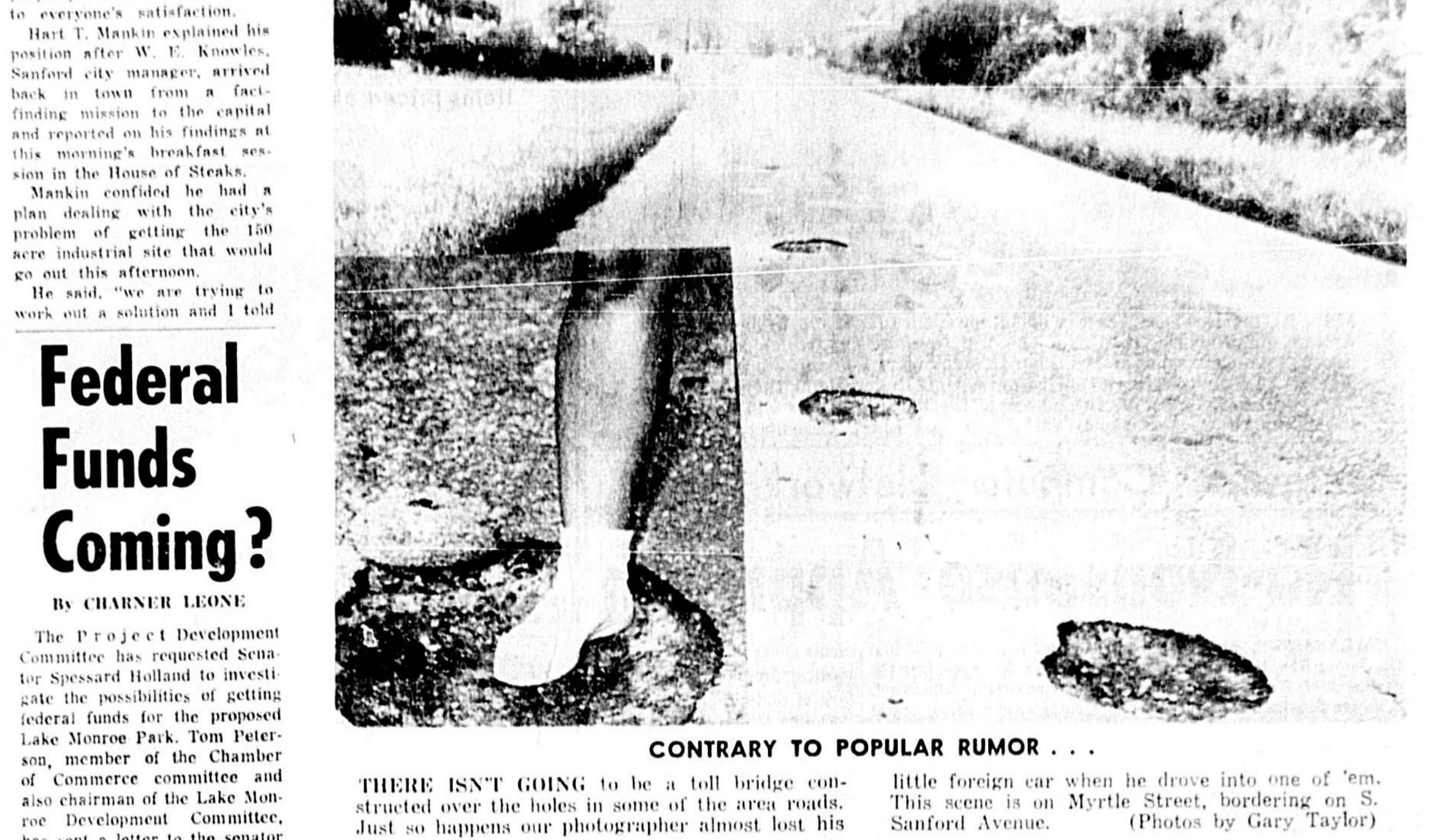
CONTRARY TO POPULAR RUMOR... THERE ISN'T GOING to be a toll bridge constructed over the holes in some of the area roads. Just so happens our photographer almost lost his little foreign car when he drove into one of 'em. (Photos by Gary Taylor)
