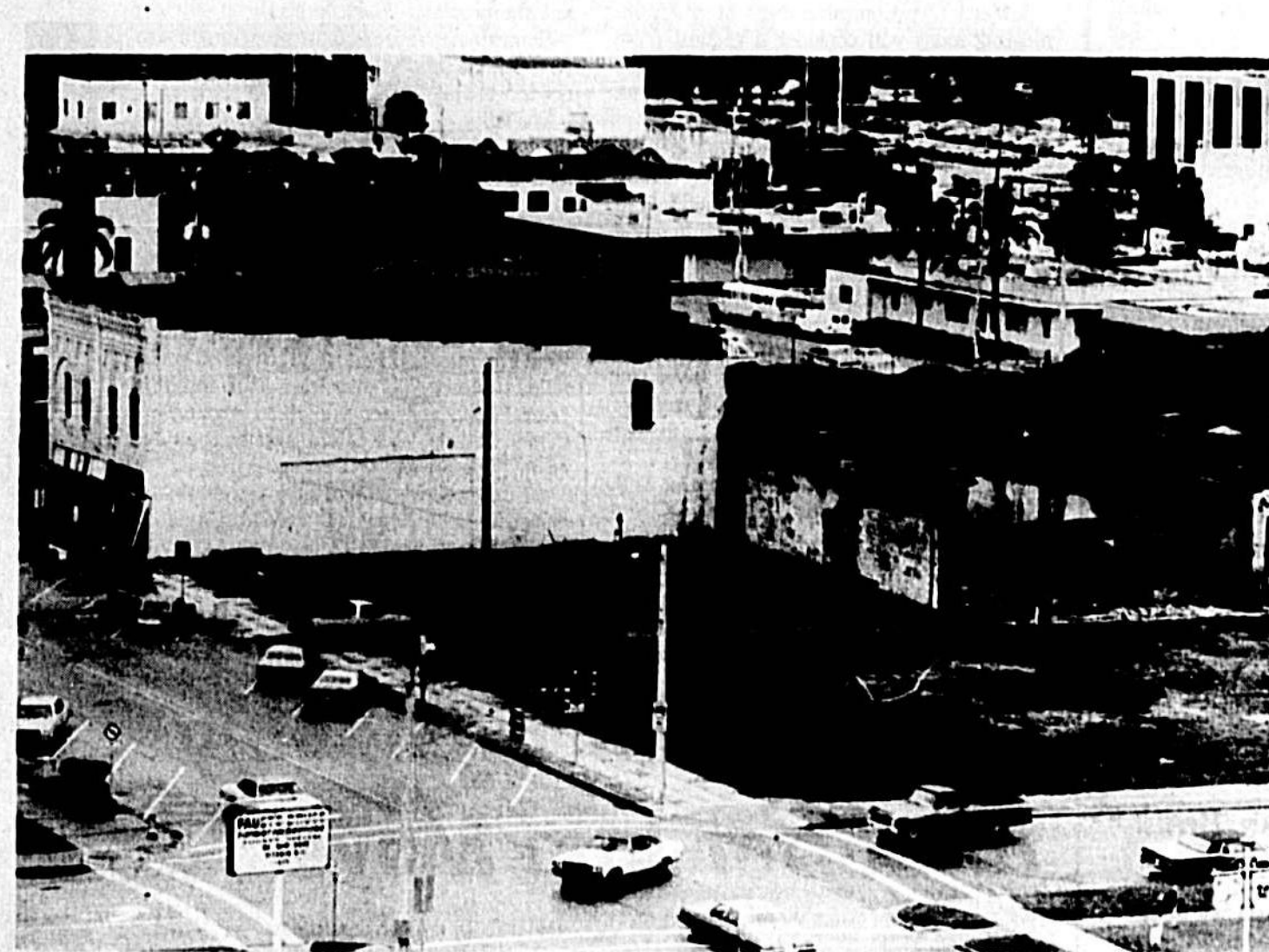
Barricades (lower left) block traffic on First Street in front of the Factory Furniture Closeouts store, which was among several buildings destroyed in a half-block area Sunday night. Fire officials will keep the markers in place until wall of the store is declared safe.
