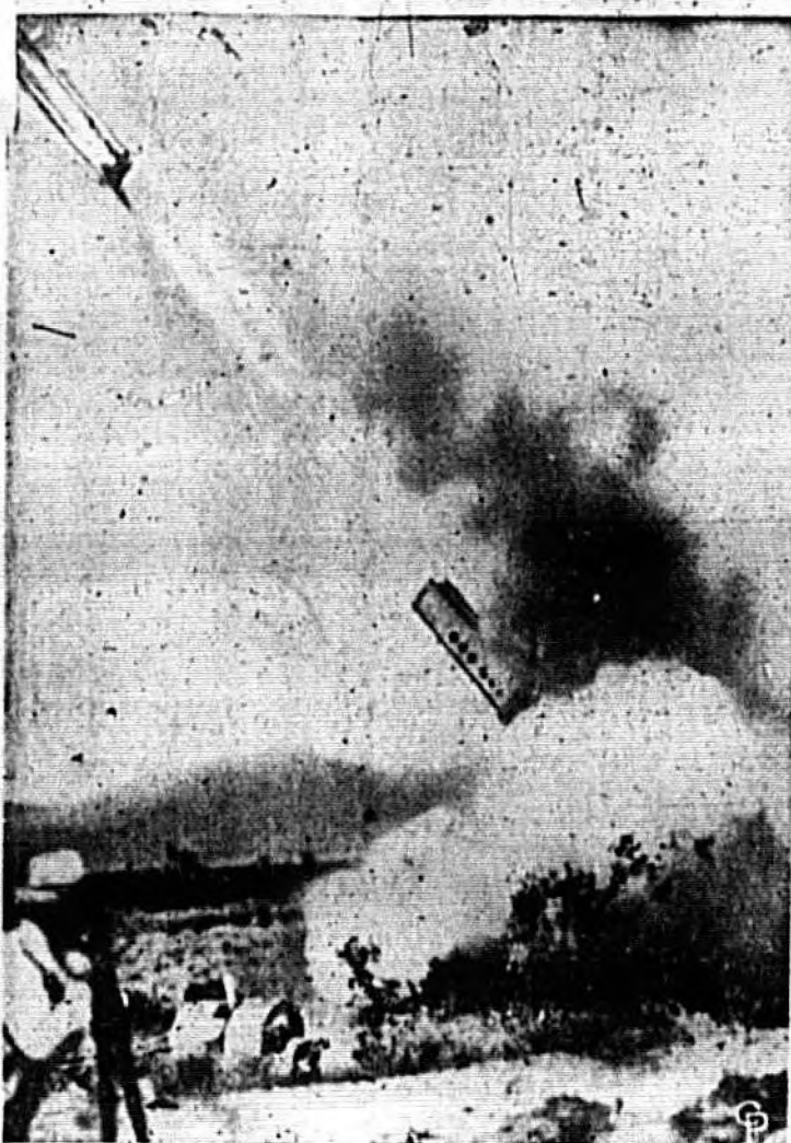
POWERED BY A JATO (jet assisted takeoff) solid fuel rocket, a radio controlled anti-aircraft missile is off for its target, during tests at Mojave, Calif., Naval Base. The Kun-2 (Little Joe) is normally launched from catapult with the aid of four standard rockets. (International)
