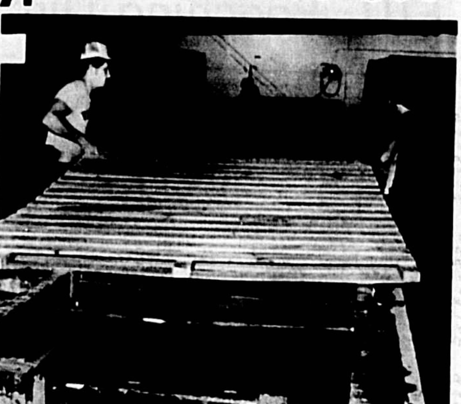
REMOVING FINISHED FENCE SECTION FROM JIG
