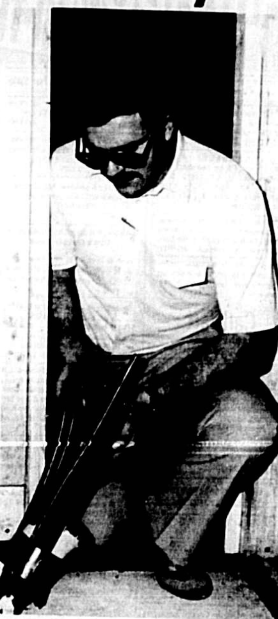
Builder Gino Ratti and connection for heat pump air conditioner.
