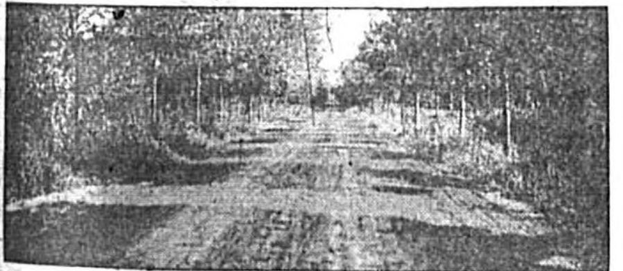
The entire 17 miles of the Savannah race course is saturated with oil.
