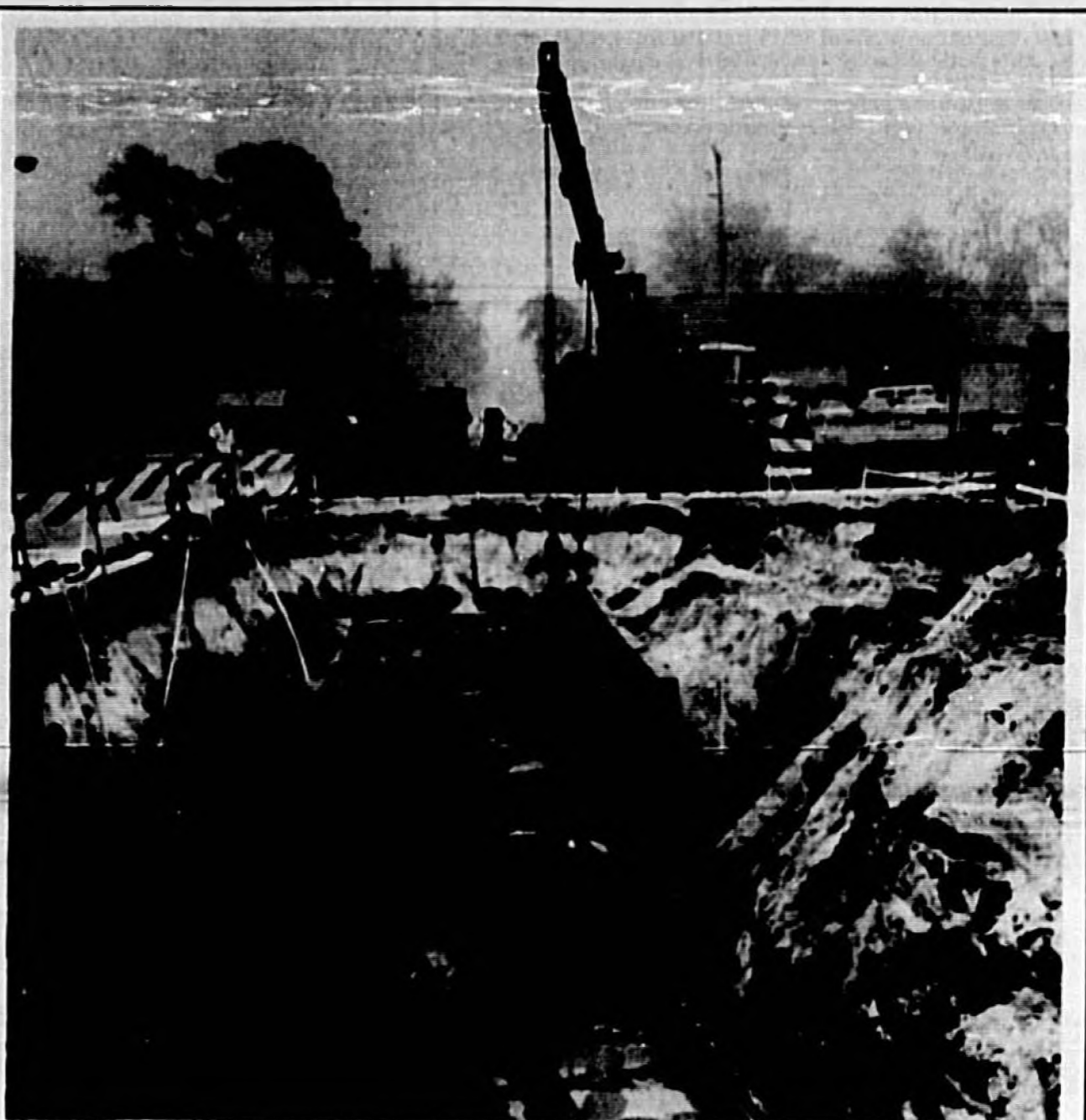
Workers began laying pipe at Mangostine Ave. and S.R. 46 last week.
