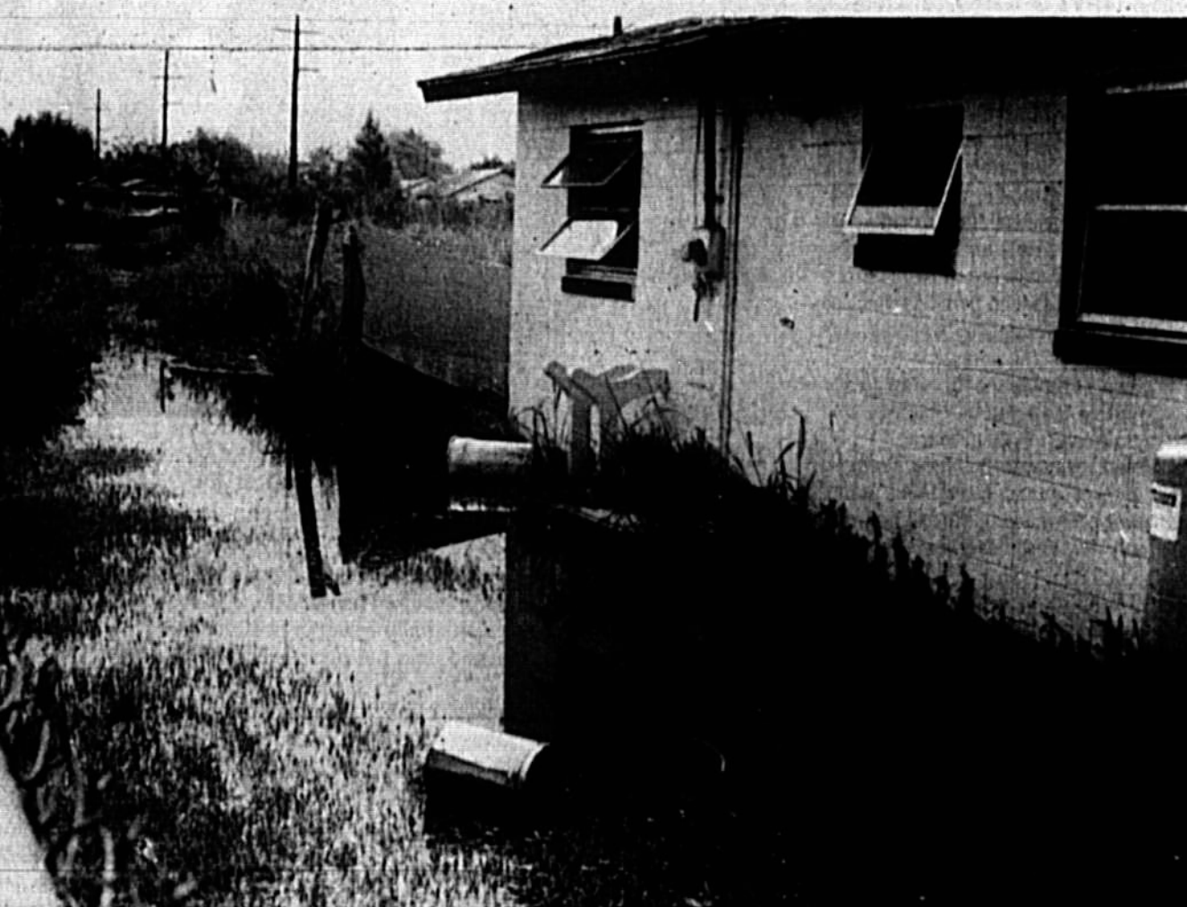
Torrential rains didn't help the Madison family on Granby Street in Midway as evidenced by the standing water in their back yard. Willie B. Madison of Rt. 1, Box 221, said the water surrounds the house and was too deep Saturday for the children to go outside. She blamed Seminole County work crews that neglect to clean area ditches for the problem.
