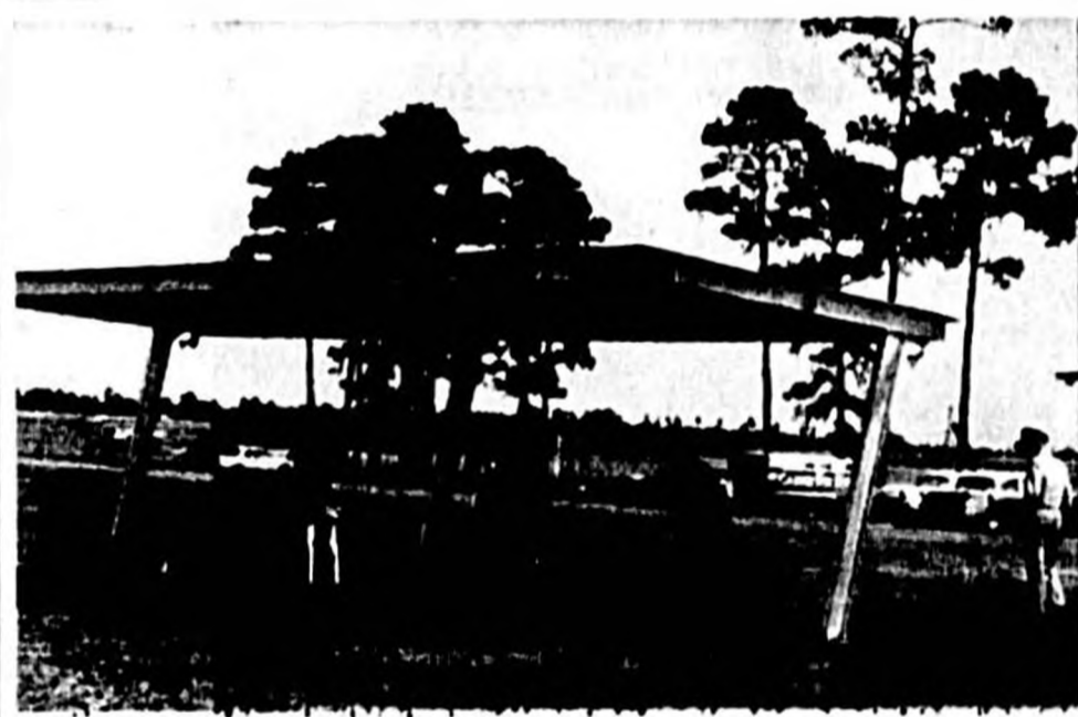
THIS GOLF DRIVING range was constructed last spring to provide recreation for the golf-minded military personnel and their dependents. It is located near Sanford Naval Air Station's Lake Golden. The facility cost almost $3,000. (Official Navy Photo)
