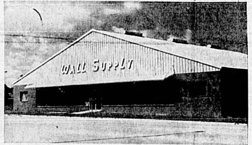
WALL SUPPLY COMPANY — An American Steel Building located on North French Avenue in Sanford, Florida — completed in record time.
