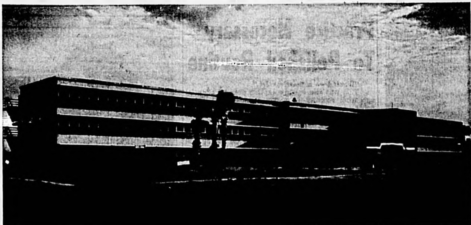
THIS 308-MAN barracks, which cost more than $560,000, was opened in August. The three-story structure, occupied by
