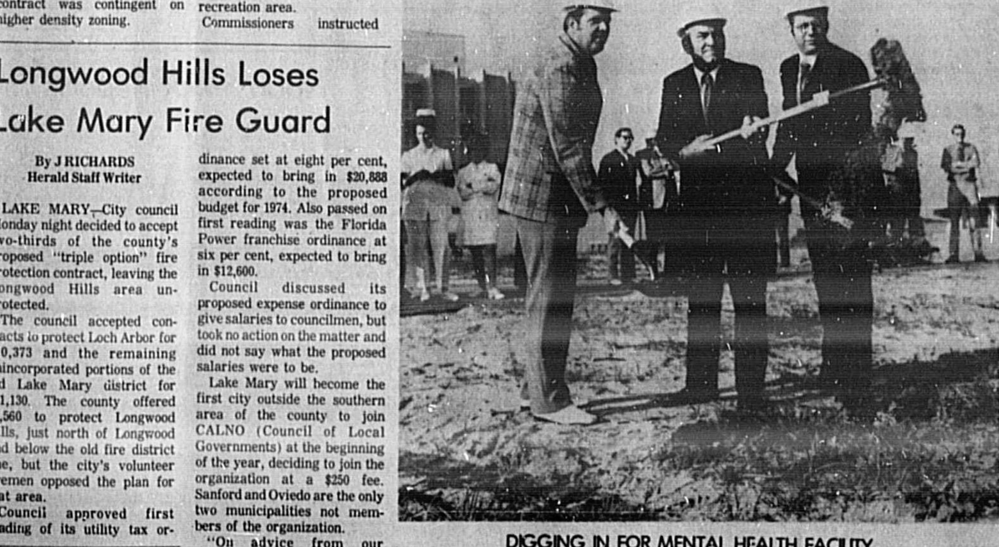
DIGGING IN FOR MENTAL HEALTH FACILITY
