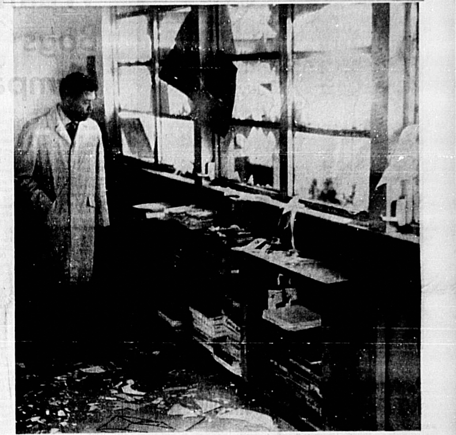
CULPRITS HAVE ALREADY BEEN CAUGHT WINDOWS were demolished at Hopper Elementary School Monday night by three juveniles using a heavy board. Charles Robert, above, school principal, surveys the scene which greeted him this morning when teachers arrived at the Celery Avenue 1-5 grade facility to begin classes. Sanford Det. Sgt. William Lykens said two of the 12-14 year-old suspects had been charged and a third is being hunted by authorities. (Staff Photo)
