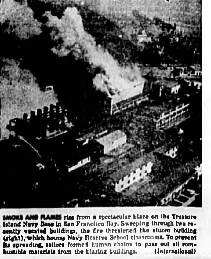
SMOKE AND FLAMES rise from a spectacular blaze on the Treasure Island Navy Base in San Francisco Bay. Sweeping through two recently vacated buildings, the fire threatened the stucco building (right), which houses Navy Reserve School classrooms. To prevent fire spreading, sailors formed human chains to pass out all combustible materials from the blazing buildings. (International)
