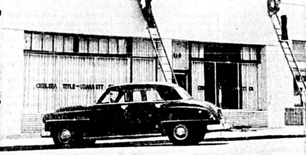
CHELSEA TITLE AND GUARANTY CO. has recently completed face lifting redecoration to the front of their First St. offices. Here workers put the finishing touches on the job by attaching letters to front of building. (Herald Photo)
