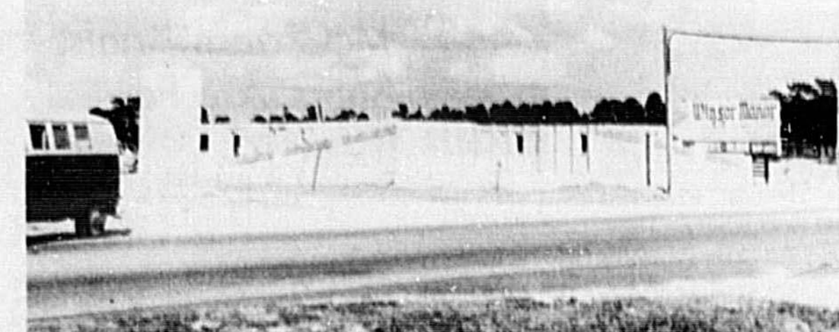
The first photo above depicts the fact that even though developers filled in the marshy flood-prone area and dug a lake to take care of the storm drainage, when there is a heavy storm, in addition to the water going to a holding pond, it goes across the highway to Island Lake (bottom). The shore line comes to the edge of the highway shoulder and the photo of the lake illustrates the degree to which the lake level has risen.
