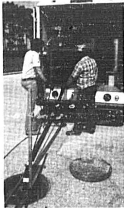
The 'sewer viewer' ...it beats digging up streets and lawns
