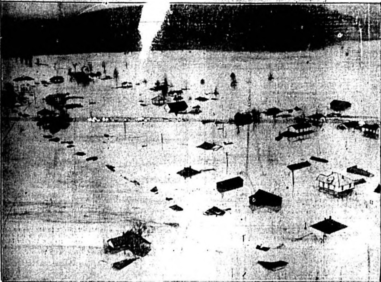
Only the house tops in Green Springs, W. Va., were in sight above flood waters when a photographer flew over and made this picture. The town was one of many swept by torrents that caused scores of deaths, drove thousands of people from their homes and wrought damages estimated at millions of dollars in eastern states. (Associated Press Photo)
