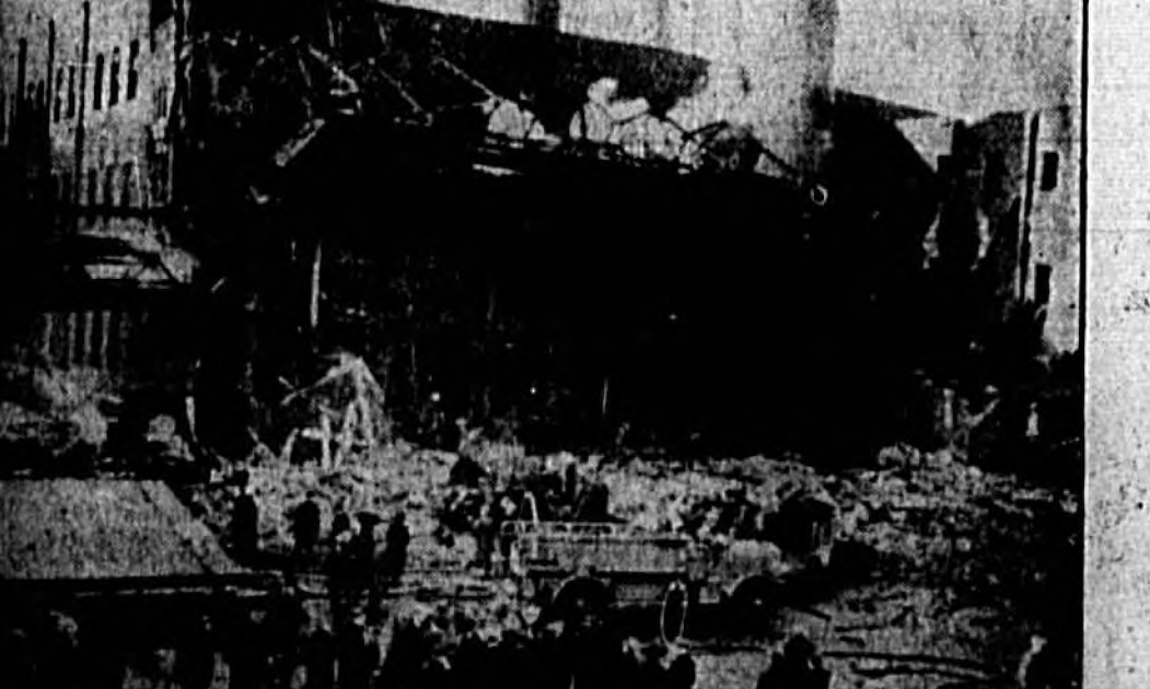
This is a view of the wreckage caused by a series of explosions in the plant of the Heaton Brewery in New York which killed four persons and injured 10 others. The blast leveled the structure in the foreground and damaged the company's main building in background.
