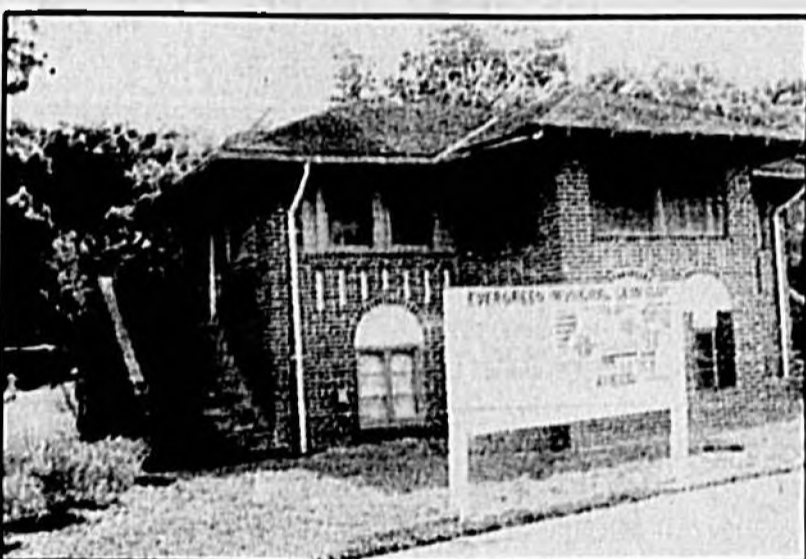
Left, the structure formerly known as the caretaker's residence at Evergreen Memorial Cemetery in Sanford, also proposed for demolition. Inspectors have discovered the building has a number of structural problems which prevent it from being within city code parameters. Along with the gazebo, the Cemetery Advisory Committee is recommending demolition.
