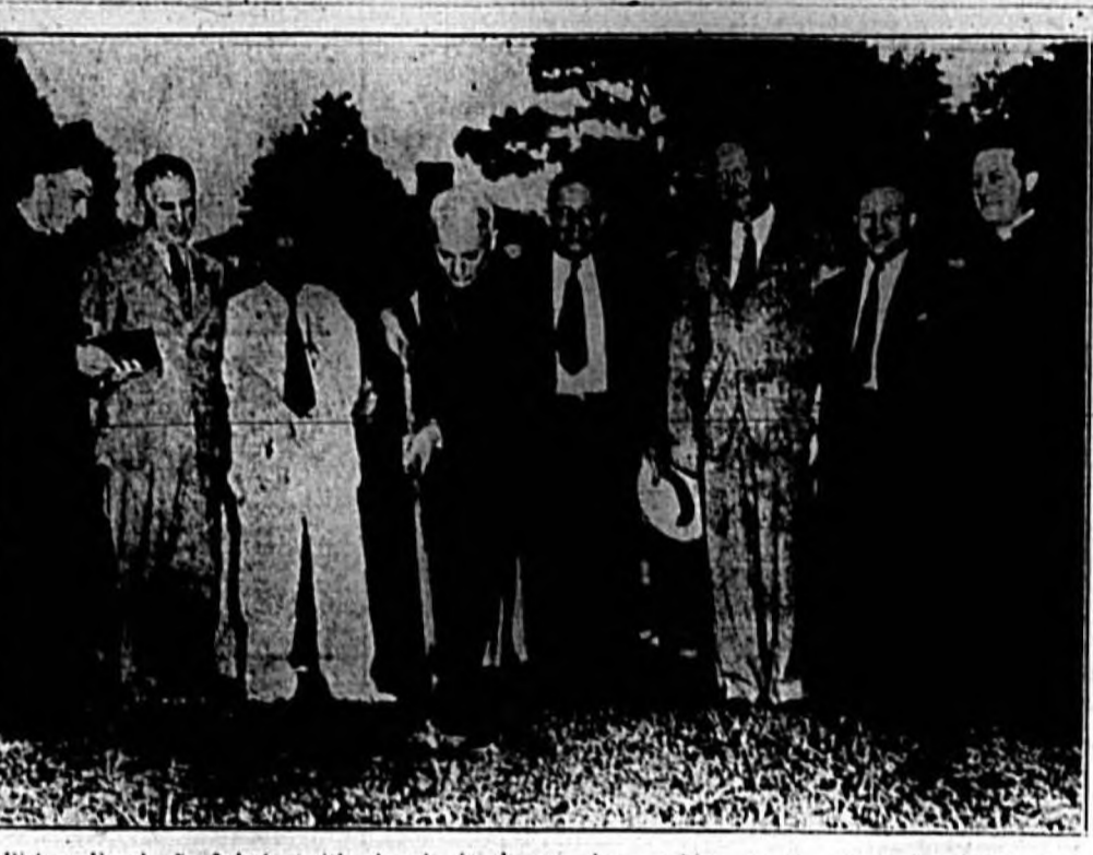
Bishop Frank A. Juhah (with shovel) is shown above taking up the first shovel full of dirt at ground-breaking ceremonies during the start of construction of the new $25,000 Episcopal student chapel at the University of Florida. Officials who participated in the ceremony are (left to right), Rev. Hamilton West, Episcopal student pastor at the University, Rudolph Weaver, director of the school of architecture and architect of the chapel, Klein Graham, representative on the building committee from the Diocese of Florida, Bishop Juhah, W. A. Shands, Gainesville, treasurer of the building committee, Dr. John J. Tiers, president of the university, Rev. Martin Bram, pastor of Holy Cross Church in Sanford and representative on the committee of the Diocese of South Florida, and Rev. Francis Wakefield, pastor of Holy Trinity Episcopal Church in Gainesville.
