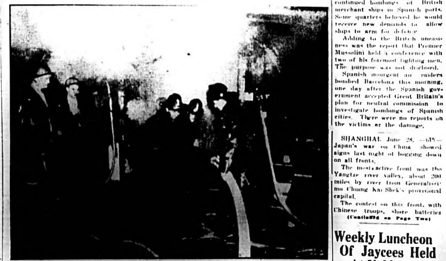
In the $54,000,000 vehicular tunnel being constructed 150 feet beneath the East River in New York, firemen are shown battling a fire that broke out in the construction timbers supporting the roof of the bore.
