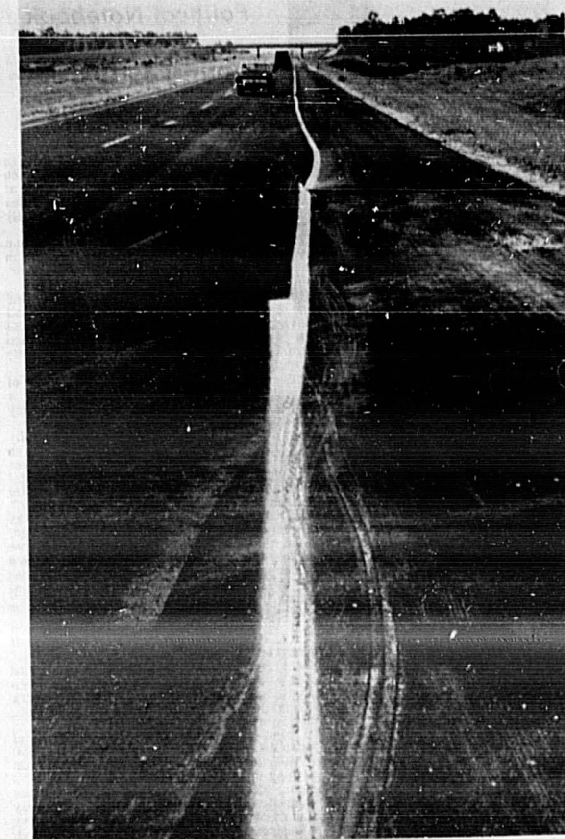
HIC! The line painting machine that did this job of marking westbound section of Interstate 4 between SR 46 and 20th Street apparently had a severe case of hiccups.
