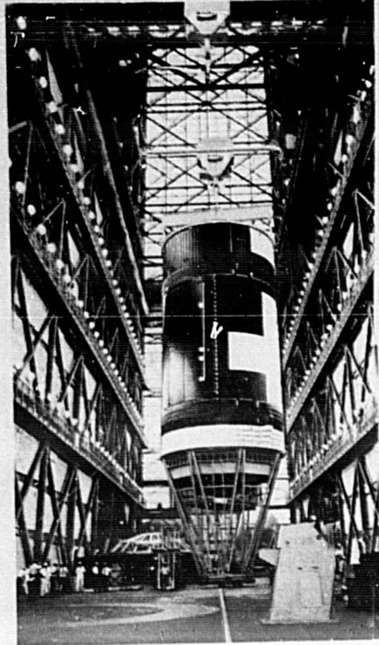
HIGH-RISE space hardware is dwarfed by the High Bay area of Cape Kennedy's Vehicle Assembly Building. Section in the Skylab Orbital Workshop which will be mated with a Saturn V launch vehicle for the Skylab mission, scheduled for 1973 launching.
