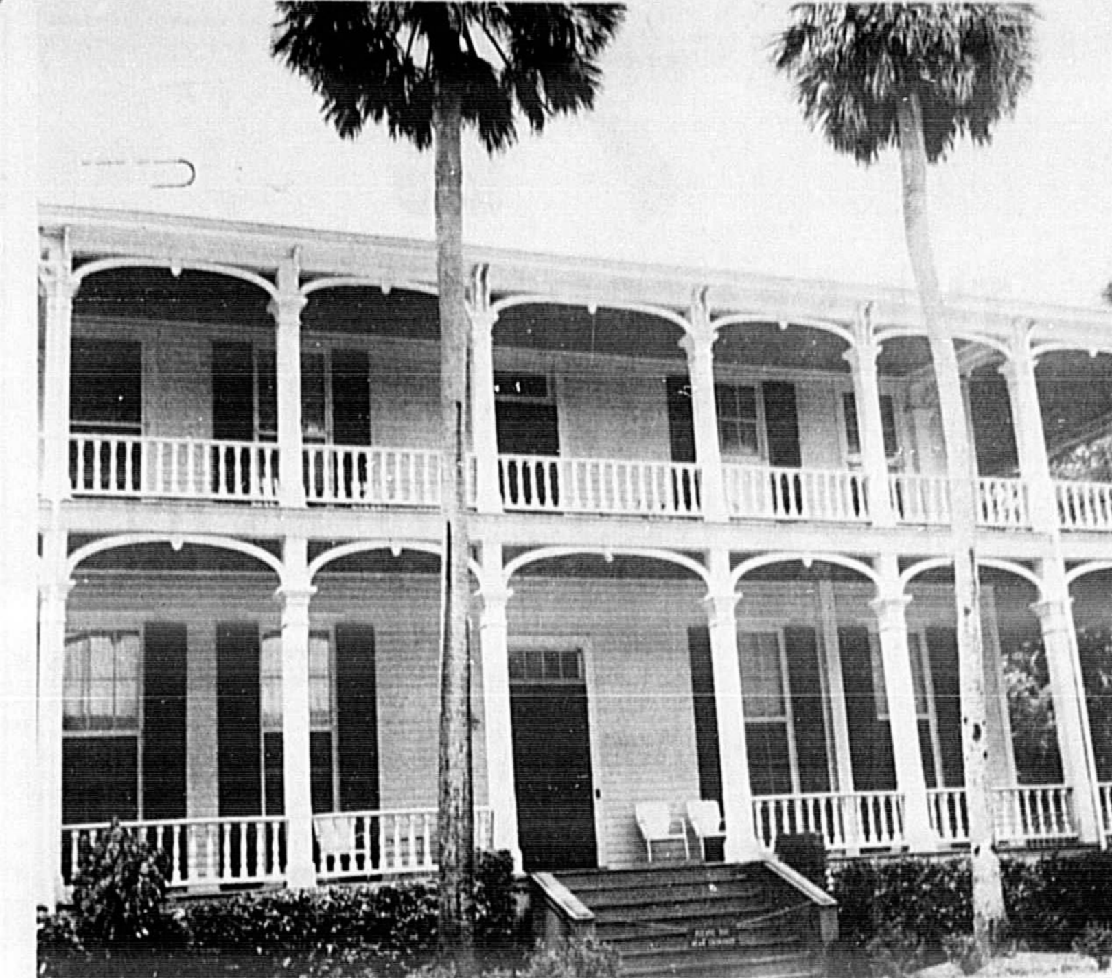
DEBARY HALL and Art Galleries is the headquarters for Florida Federation of Art and is open to the public everyday except Monday, 1-5 p.m. The historic mansion was built in 1871 by Count Frederick DeBary, a German of Belgian descent, after whom the modern day community of DeBary was named. (Carl Allen Photo)
