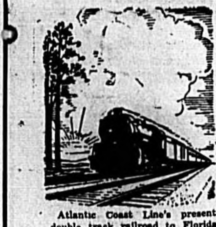
Atlantic Coast Line's present double track railroad to Florida.
