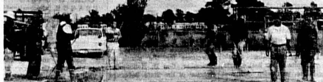
WORK has begun on the project of the County Commission to provide county-wide recreation facilities at neighborhood schools. Commission Chairman John Alexander (top photo) inspects finishing stages of the new tennis court at Orisno School, Ball Field at Wilson School (center photo) is already completed and being used. Men of the county crews finish concrete (bottom photo) on the hard surface utility court at Longwood School. Value of the facilities, when work is completed at all schools over the next three years, has been estimated at $100,000. (Herald Photos)
