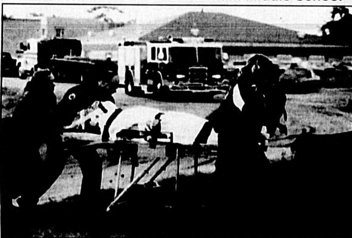
A worker for Southern Fire Protection in Sanford was injured 9:16 a.m. Friday at Millennium Middle School when a piece of lift equipment he was on became unstable. The lift equipment shifted under the worker, who has not been identified, and tipped over, causing the man to fall. He was transported to Orlando Regional Medical Center as a precaution, according to a spokeswoman for the Sanford Police Department.
