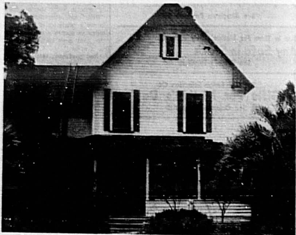
THE FORMER Enoch Partin home recently purchased by Mr. and Mrs. Tom Bowers will indeed be a show place once again when Tom Bowers completes his renovations. The home was built in 1859 and is the former residence of Mrs. Lucille Niblack and her brother James Partin. There are eight rooms and Bowers is doing all of the work in his "spare time." Mrs. Bowers, Essie, is a surgical nurse at Orange Memorial Hospital and they have four children, Tim, Ted, Tod and Tammy.
