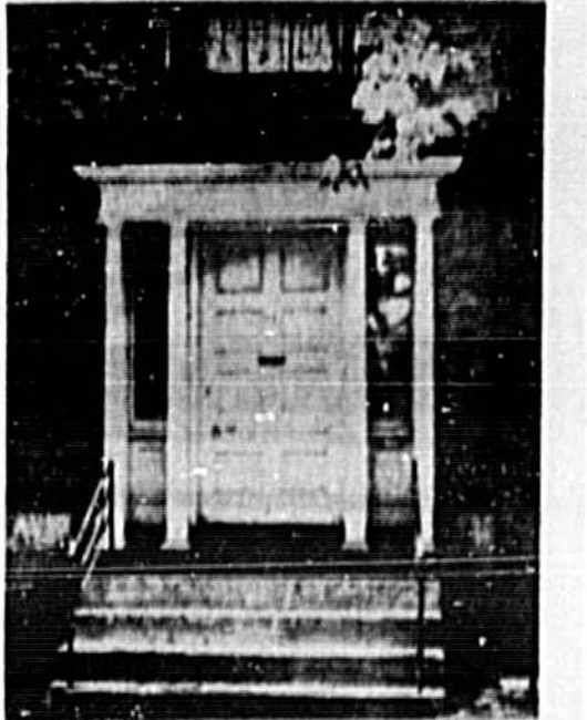
THIS 1806 DOORWAY photographed on Boston's Beacon Hill was designed by renowned architect Charles Bulfinch. The drawing shows a contemporary version, factory-made of ponderosa pine. The new unit retains the carefully scaled dimensions and authentic details of the early American entranceway.
