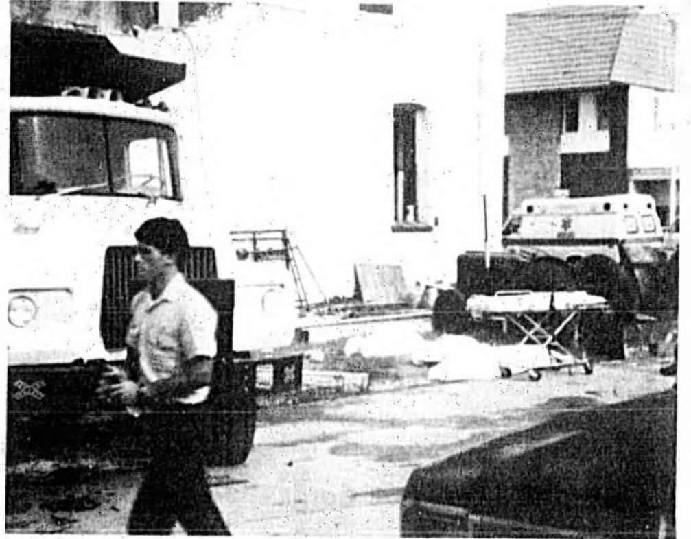
The bodies of the men who were killed Friday lay covered outside the west wall of the W. Atlee Burpee Seed Co. building, 206 W. First St., Sanford, shortly after the top of the two-story brick wall collapsed and fell on them. This photograph was taken by Henry Longwell who had worked for the seed company for 40 years.
