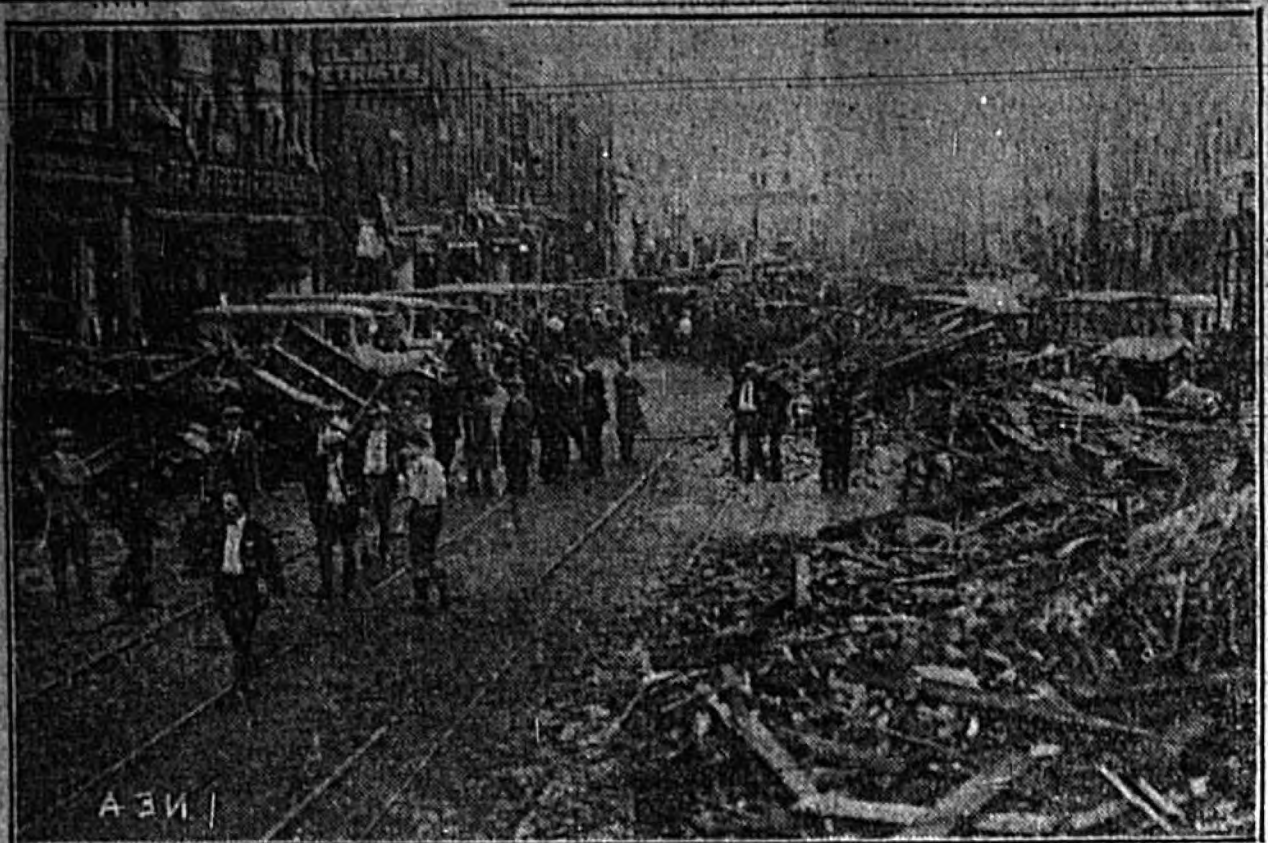
Ruins in downtown district of Lorain, Ohio, looking down Lorain's main street at dawn Sunday. Scores were buried in the debris when this photograph was made.
