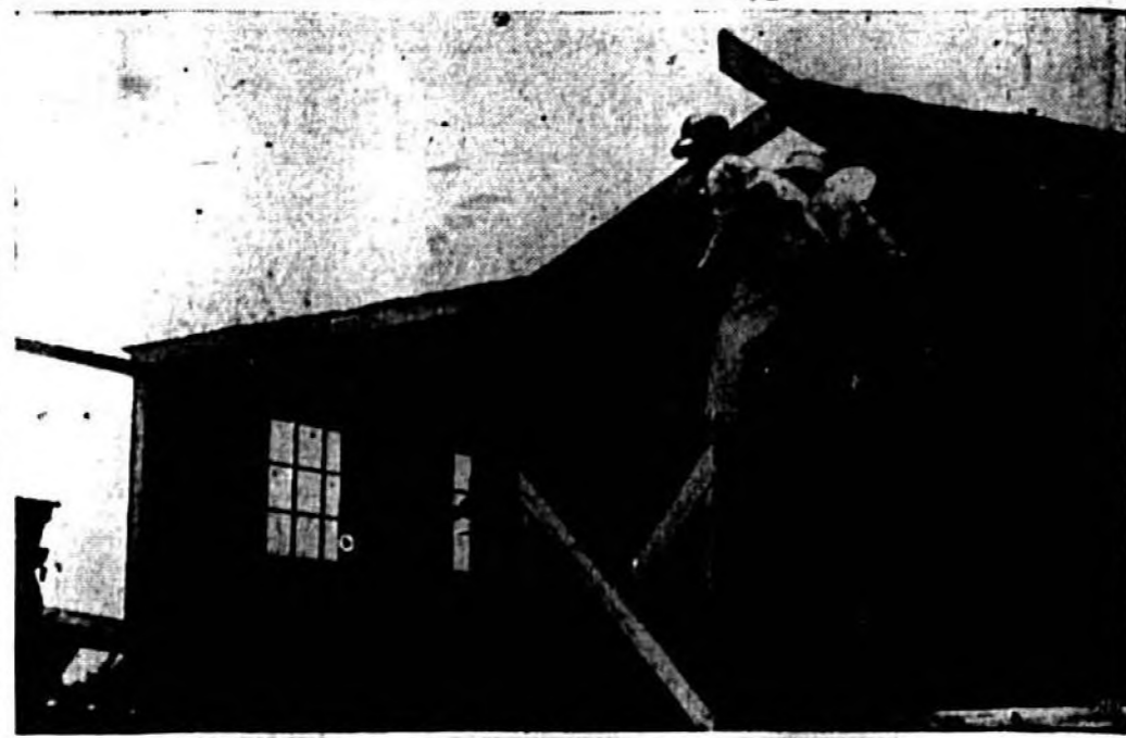
NO FOOD WAS SERVED in above mess hall being dismantled with rest of $20,000 CCC camp near Odesa, Del. Camp, built in 1925 for mosquito control program, wasn't used.
