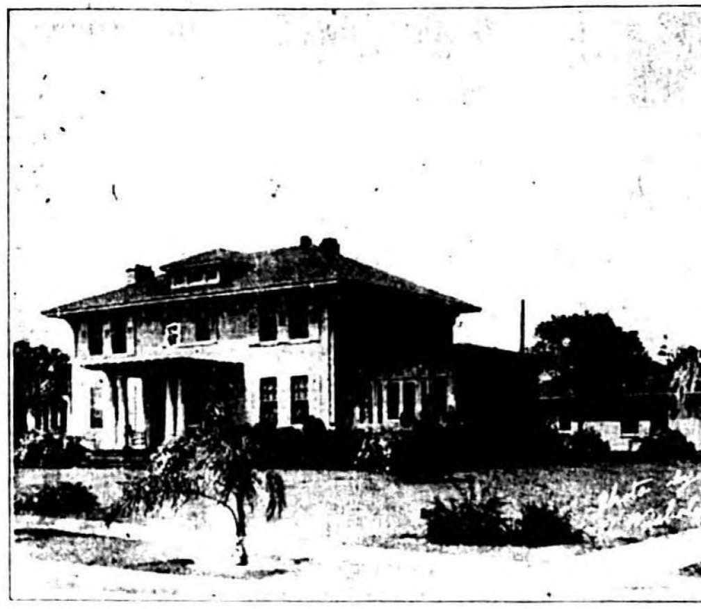
This residence, 1900 Magnolia Ave., is one of the most attractive in Sanford. It was constructed by Mr. Hill in 1924 and has since been occupied by him and his family.
