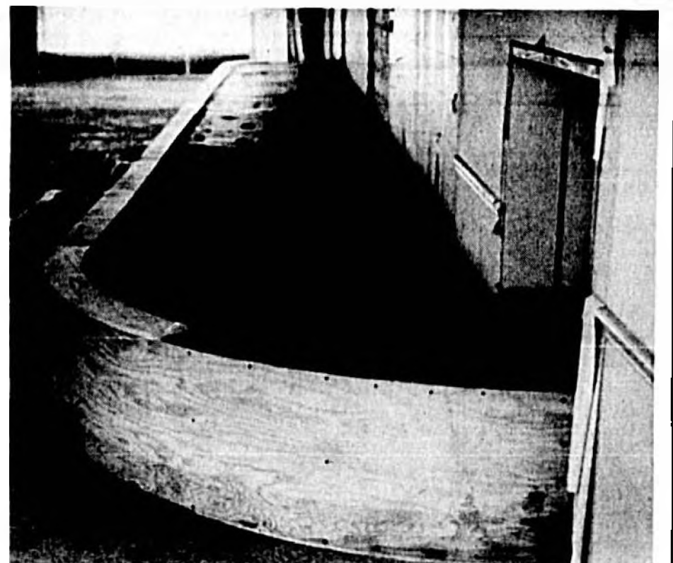
Improvements include a belt conveyor for luggage.
