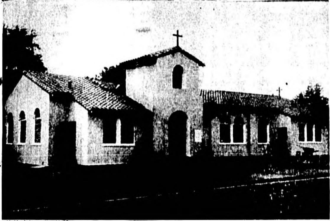
CONGREGATIONAL CHURCH—The new Sanford Congregational Christian Church is shown from its southeast corner. The edifice is of Spanish mission type architecture...
