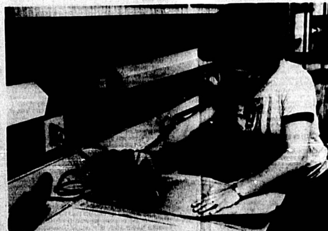
4) WAX IS REMOVED BY IRONING BETWEEN SHEETS OF PAPER TOWELS
