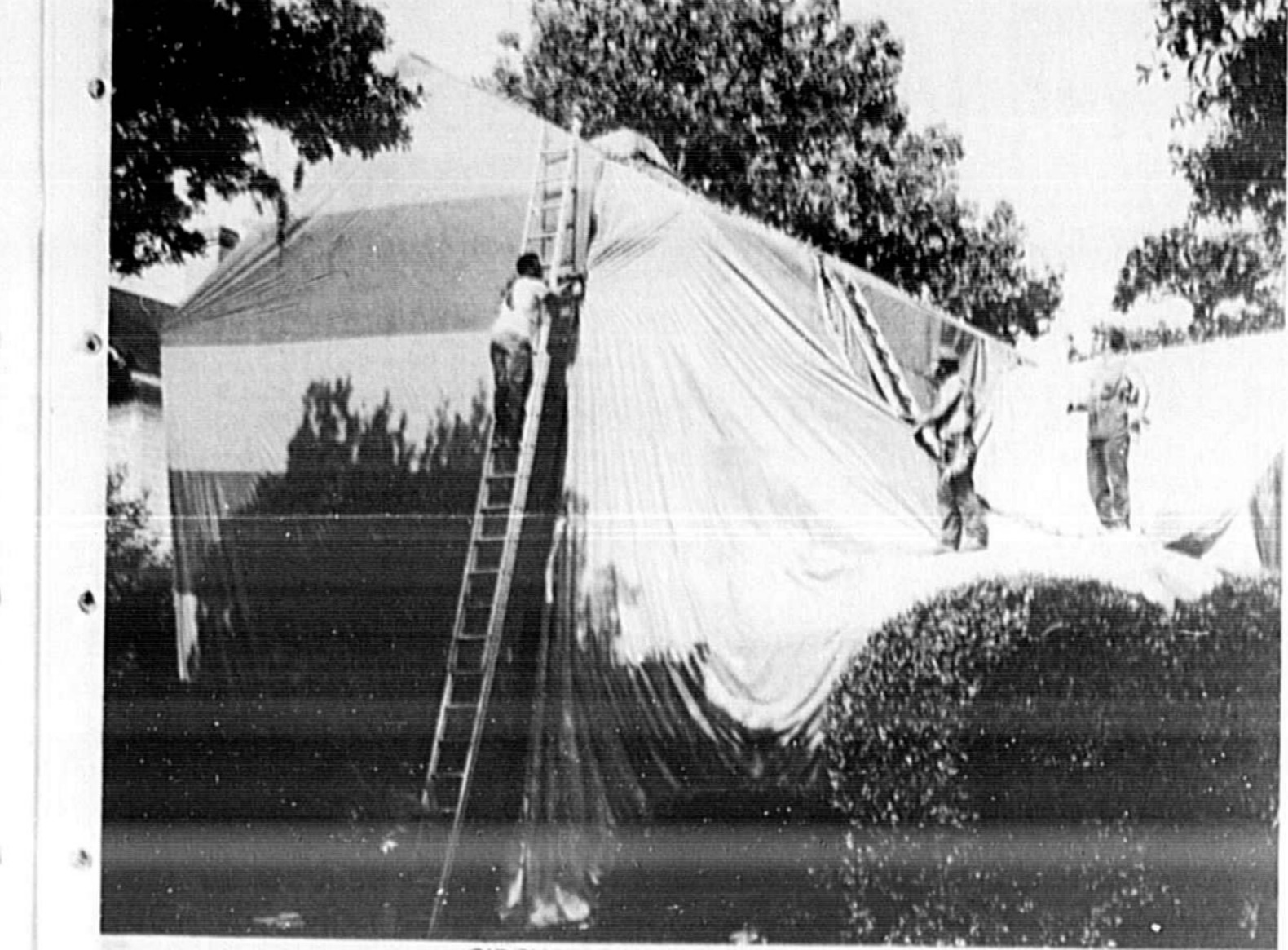
IT MAY LOOK AS IF they're setting up the Circus Big Top, but these men are not dealing with lions, tigers and performing elephants. It's the creepy-crawly animals they are after, the termites and roaches. They are a pest exterminating crew sealing a Sanford house under a giant canopy net to pumping in the pesticide.
