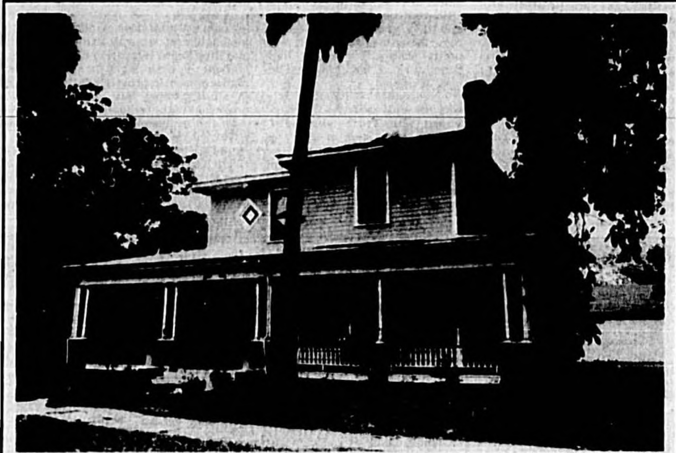
This home at 717 Park Ave. will be on the tour.
