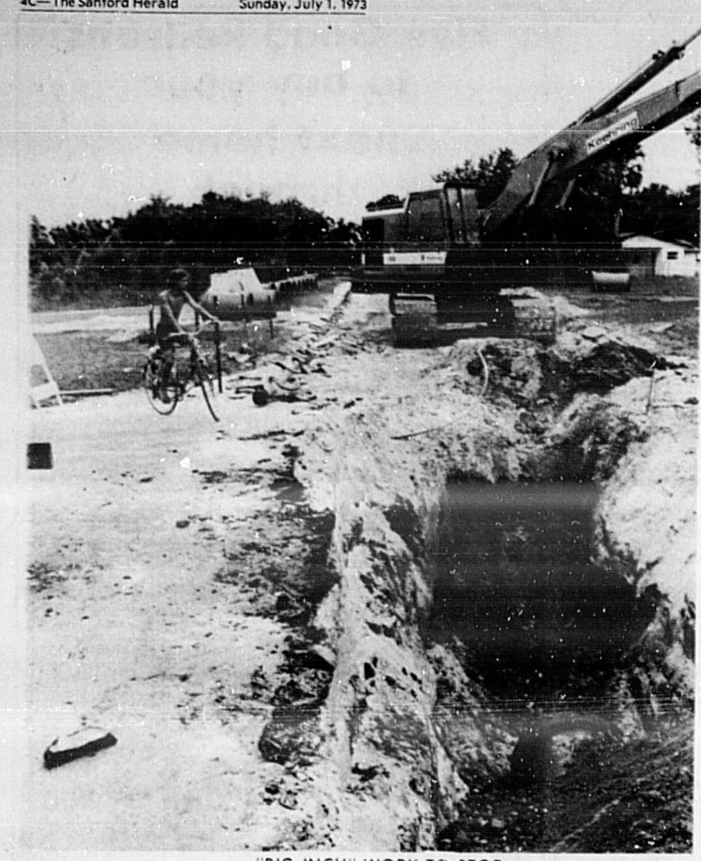
'BIG INCH' WORK TO STOP Poplar Avenue at West Third Street. After pipe sections in background are installed the project goes west and then south along an old railroad right-of-way. The "Big Inch" will link over 5,000 living units planned or under construction in the city's southern sector with the sewage treatment plant on Lake Monroe. (Herald Photo by Bob Lloyd)
