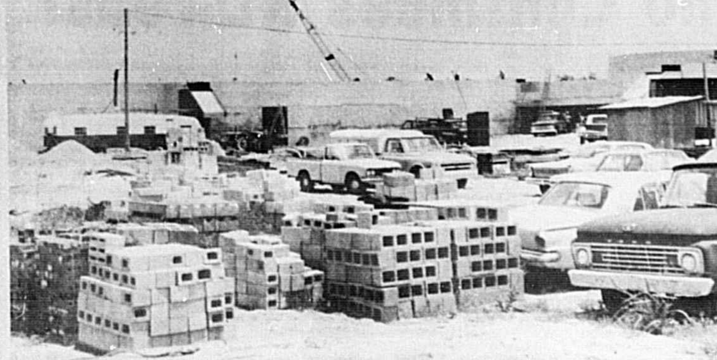
LAKE BRANTLEY High School is under construction on Sand Lake Road, Forest City, in a three-school complex which also includes already open Forest City Elementary School and Teague Middle School. The Lake Brantley facility is scheduled to open in January, 1973.
