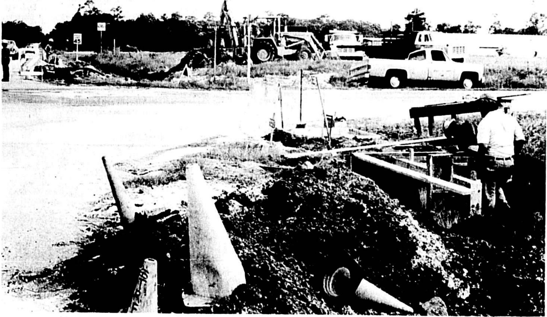
INTERSECTION WIDENED Work crews have begun widening the intersection of County Road 46A and Airport Boulevard. Ultimately, a traffic signal will be installed there, and four turning lanes will be constructed. The intersection has been the site of several major traffic accidents. Only two-way stop signs have been posted until now. (See Editorial, Page 4A).
